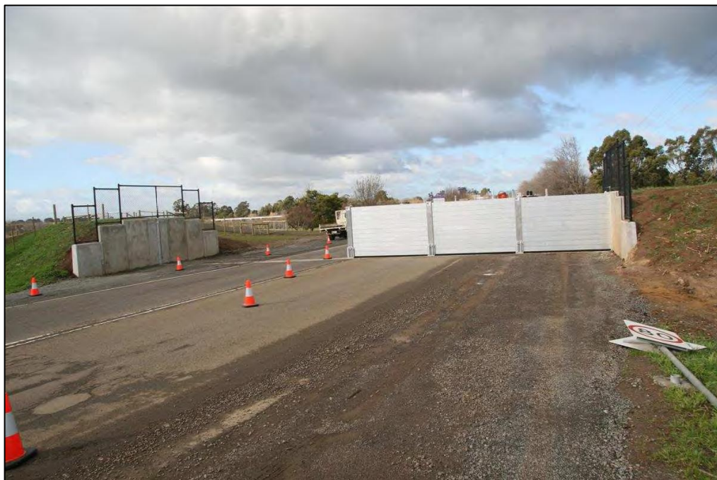
Figure 2: The BAUER-IBS DEMFLOOD System used to bridge levee gaps across roads
