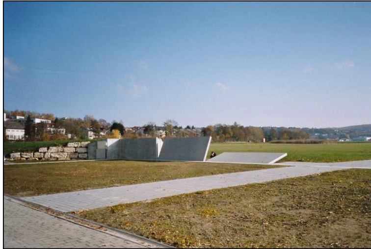
Figure 2: Completely preinstalled stationary flap system in Sinsheim near Heilbronn, Germany
