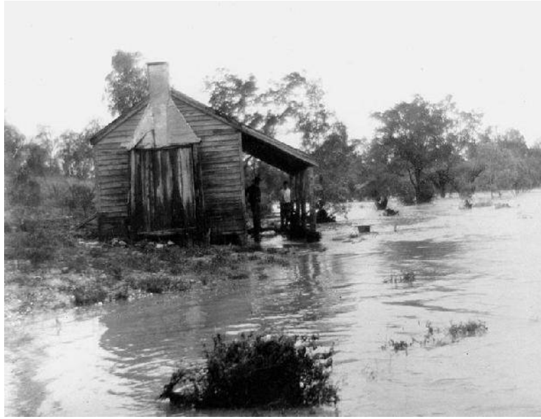
House flooded by the Barcoo River, 1906. Rough, timber house affected by the Barcoo River. Two men stand under the awning as the water encroaches upon the property. 4 February 1906 John Oxley Library, State Library of Queensland
