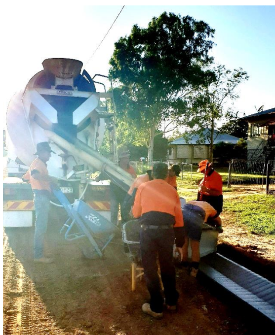
Kerb & Channel – Rose Street
