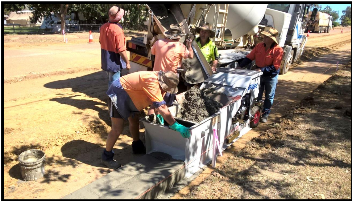
Town Street Widening and Kerbing Channel
