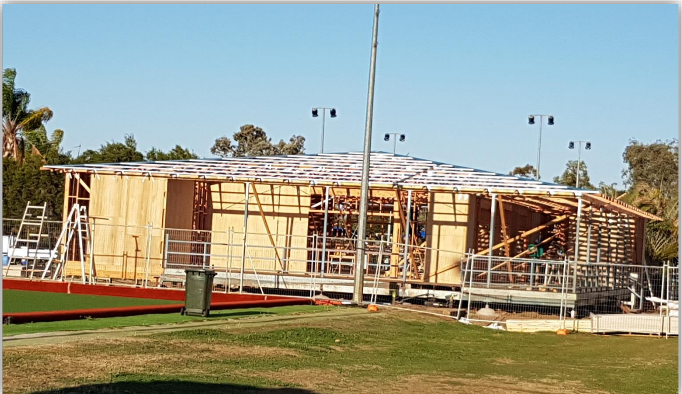
Construction of the Tambo Sports Club
